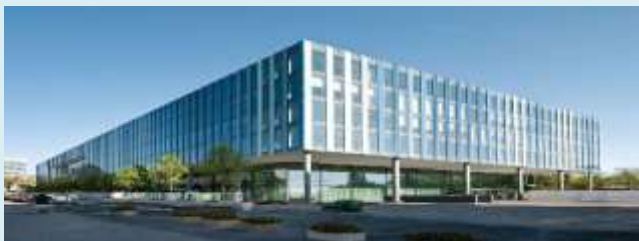
MU2-55 THE TOWER ADMINISTRATION BUILDING
